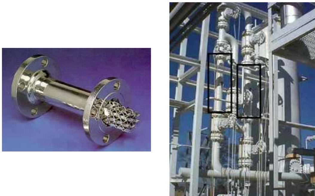
Figure 2. Static Mixer Before and After Installation.
