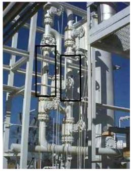
Figure 2. Static Mixer Before and After Installation.
